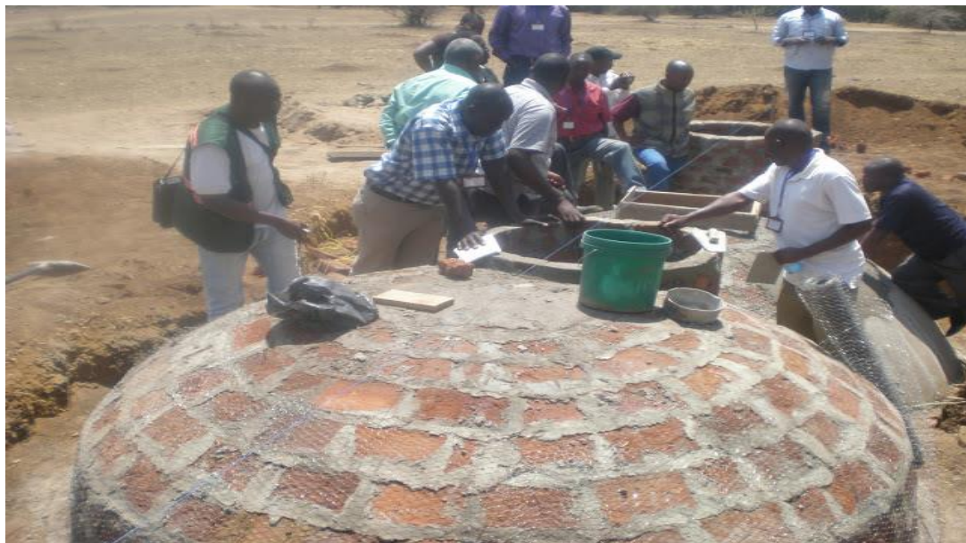
Figure 3.4: Biogas Plant Construction in Tanzania
